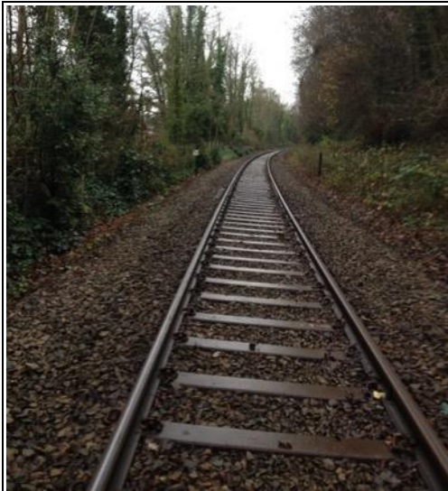
Photo 7. Portbury Fright Line Date: December 2015
