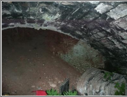
Photo 17. Pill Station arch Date: September 2016
