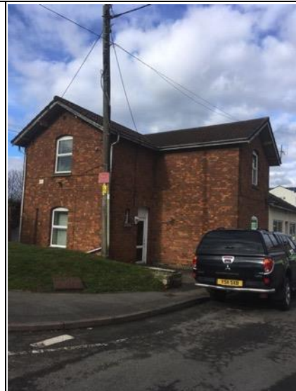
Photo 16. Station House Date: March 2018
