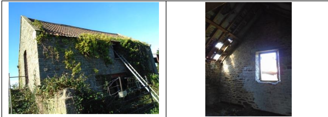
Photo 23. Lodway Farm Building LF1 – the exterior walls are solid and without crevices. Date: October 2018 Photo 24. Lodway Farm Building LF1 – the interior is exposed but internal walls are well pointed. Date: October 2018
