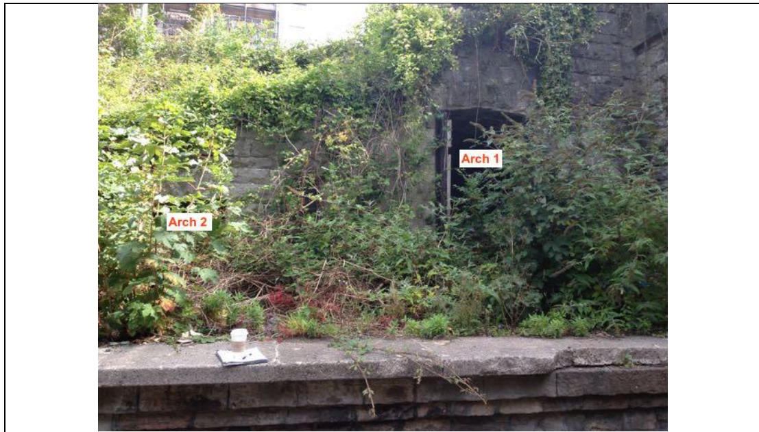
Plate 1. Arches on Pill Station Platform
