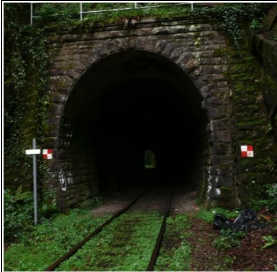
Photo 13. Railway tunnel (Sandstone) Date: November 2016
